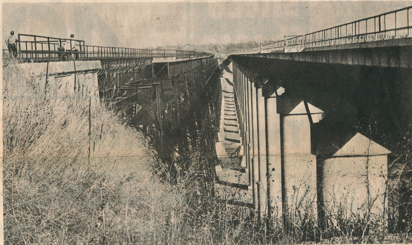
This photo shows the finished railroad bridge as it looked upon completion back in June of 1973. The old railroad bridge, eventually destroyed by DEMEX Co. of Oklahoma is shown in the background. The new bridge is composed of 22 piers and is 120 feet high. About 45 men were used in building the structure.
